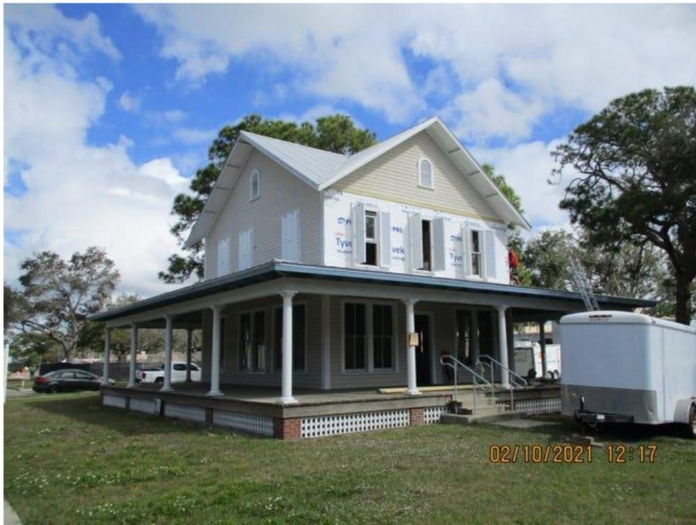
The work that Ball Construction started the week of Feb. 8 involved replacing the siding on the second floor, to stop leaks.
